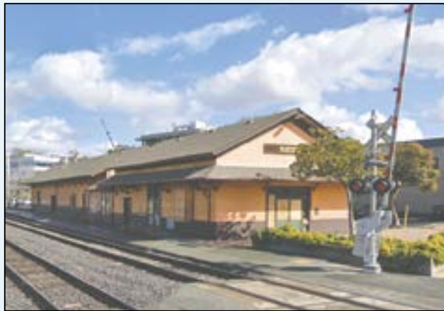
Martinez Train Depot. (Photo by Google Maps)
